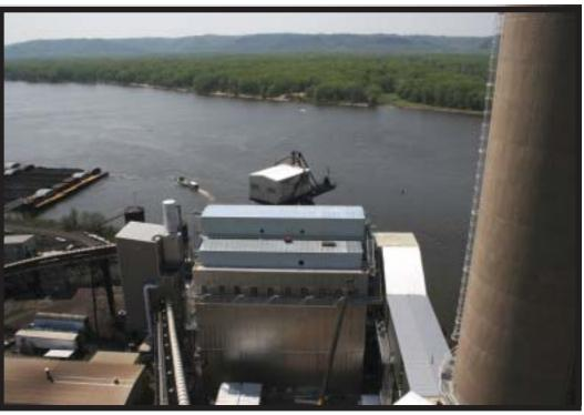
A "baghouse" (at the center of the picture) was recently installed at the John P. Madgett power station to enhance particulate matter capture.
